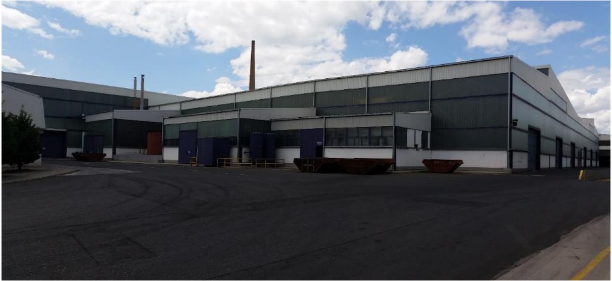
Zinc – coating Plant for Pipes
