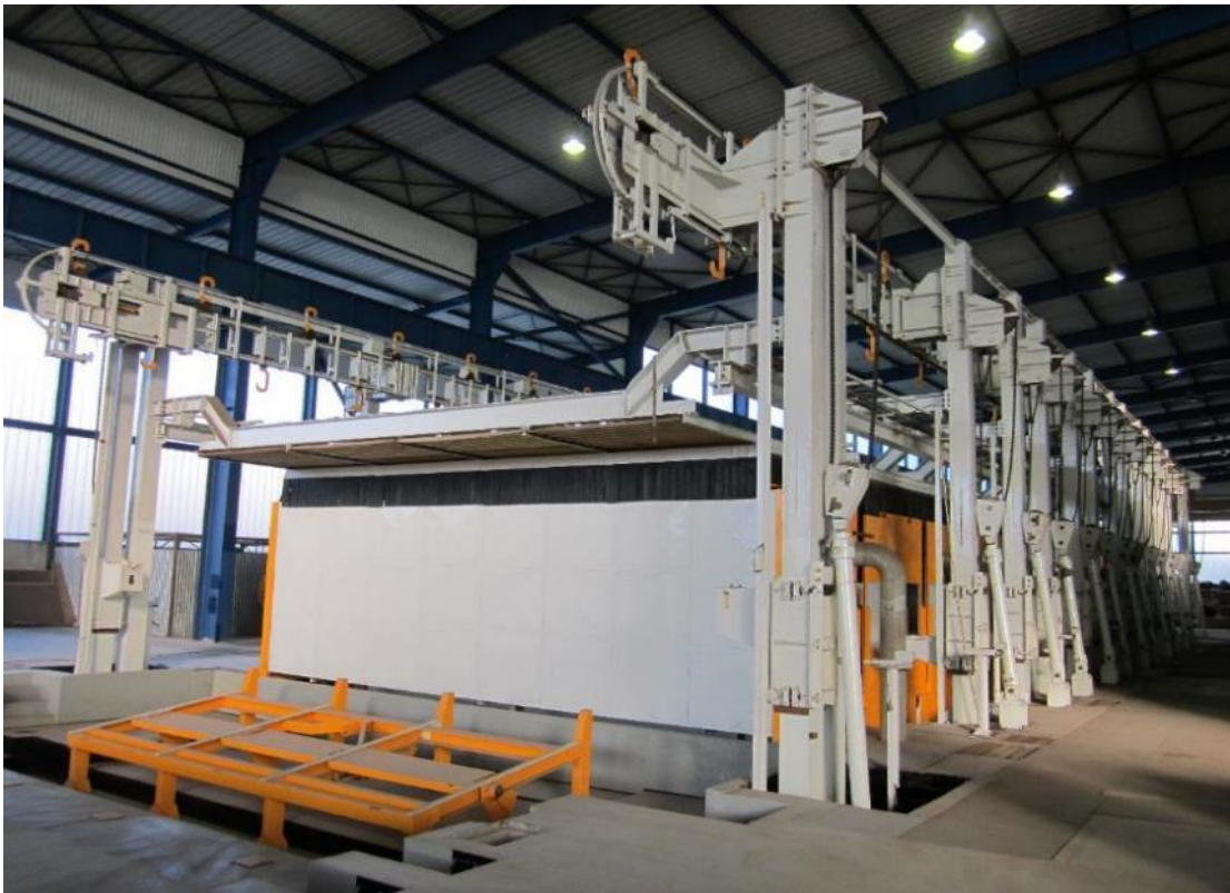
Chemical pretreatment - Exit section
