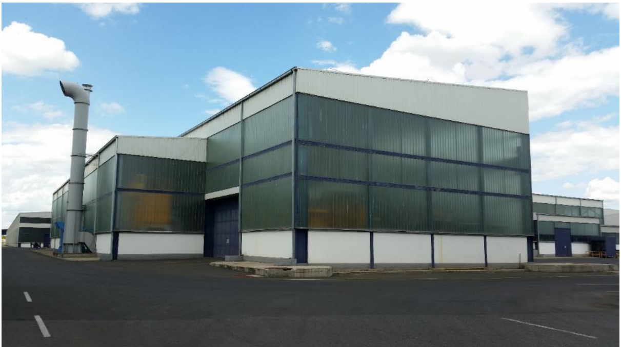
Zinc – coating Plant for Pipes
