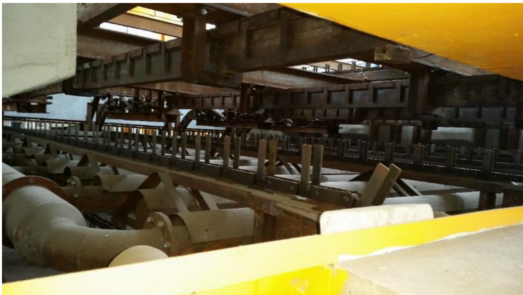
Pipe dryer - Transporters
